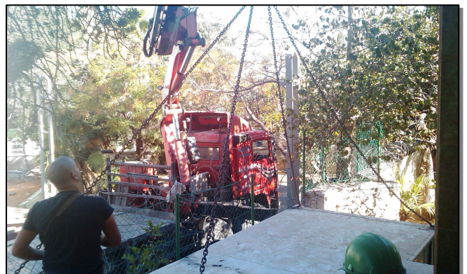
Preparing the ground: Removing the maintenance container
